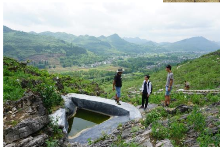
Rainwater harvesting irrigation system 集雨灌溉系统
